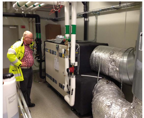
Technician Björn Adler inspecting a GOLD air handling unit. Photo: Swegon
